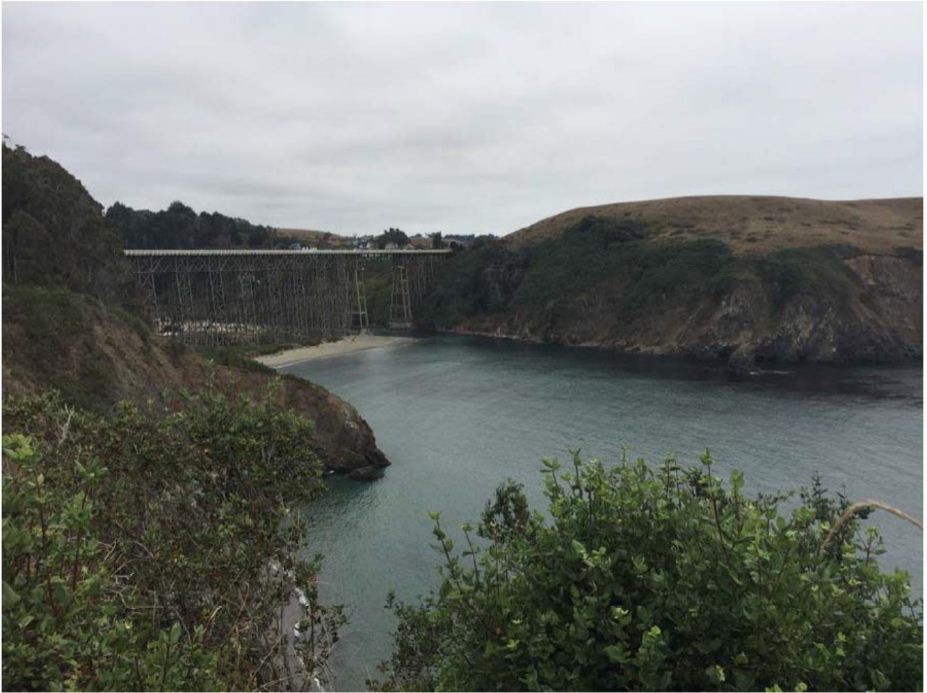
Albion River Bridge as Seen from the Albion River Inn (Looking South)
